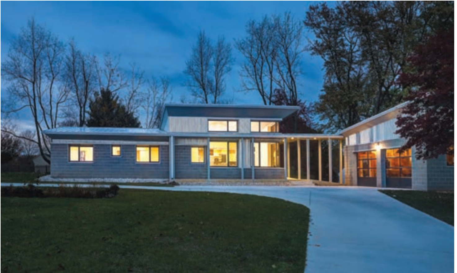
Residential Honor Award for Old Hopkins Road House: Miche Booz Architect. PHOTO: JEFF WOLFRAM
