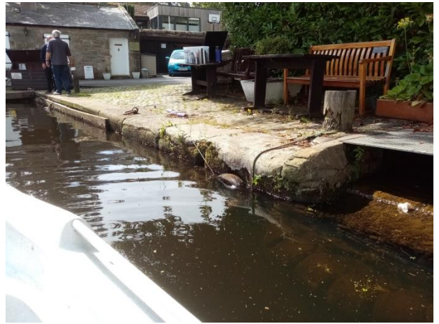
Image 4 ~ Missing Fender on West side
