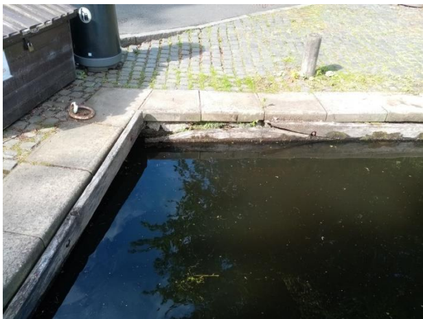
Image 1 ~ Damaged Corner Pieces
