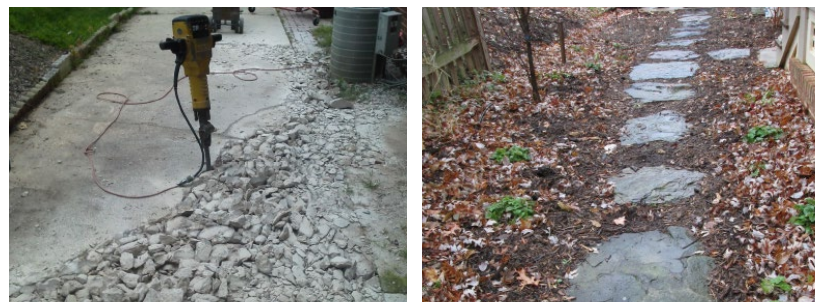
Pavement Removal
