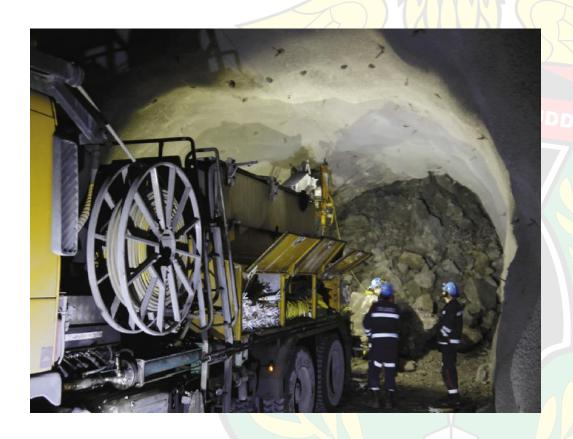
A truck loading emulsion explosive into blastholes in Kiruna underground mine
