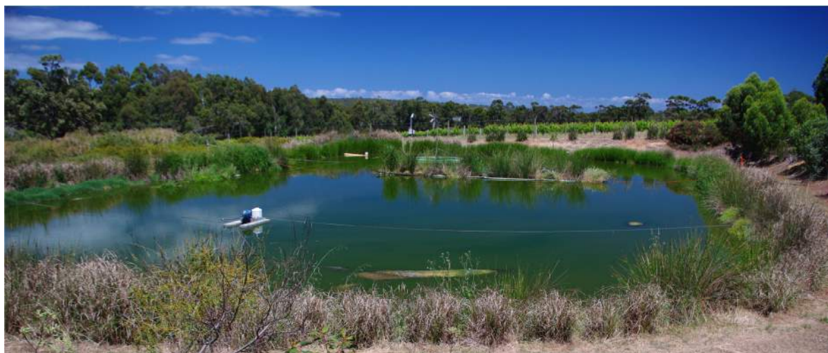
Photo 27: The combination of constructed wetland and polishing aerobic biological tank with floating islands planted by macrophytes vegetation
