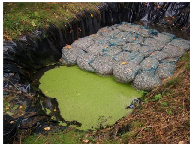
Photo 9: Example of Using Removable Sorbent Packed in Jute Sack
