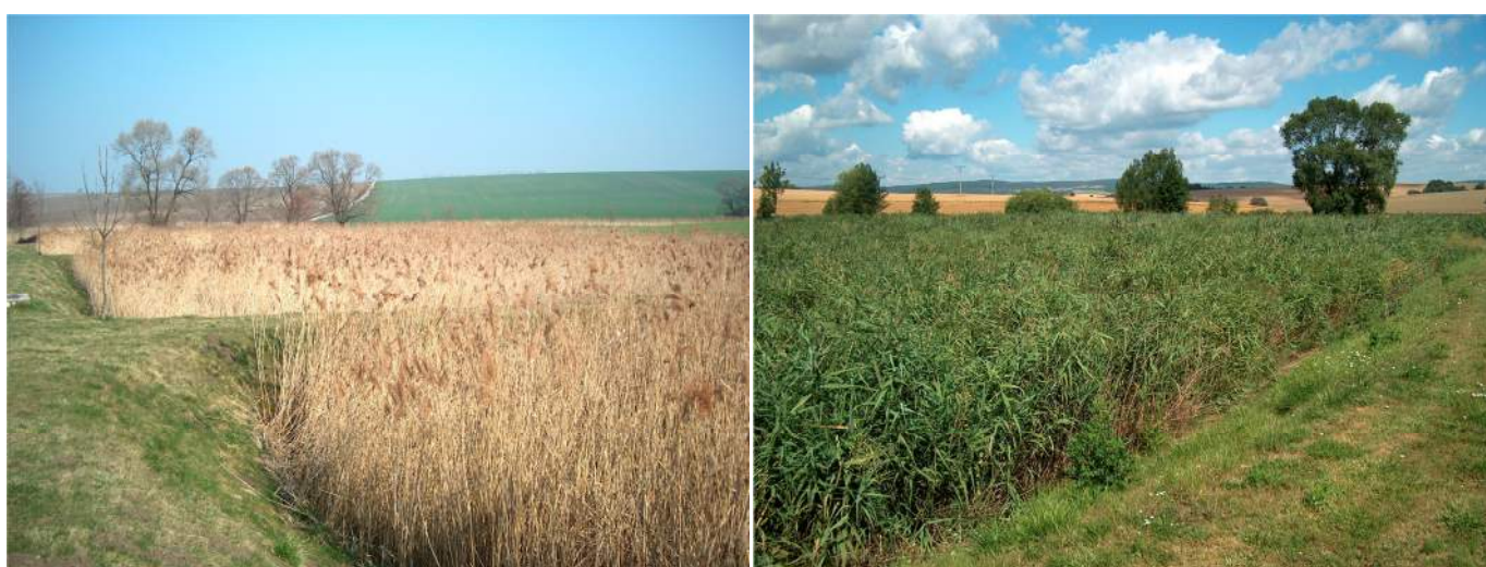
CTW at Dražovice (CZE) – Vegetation of reed is not mown, harvested or burned – a view of vegetation during the spring period at the time of sprouting of new shoots of reed (left) – a view of constructed wetland filters with high-grown vegetation of reed in the middle of the growing season (right)
