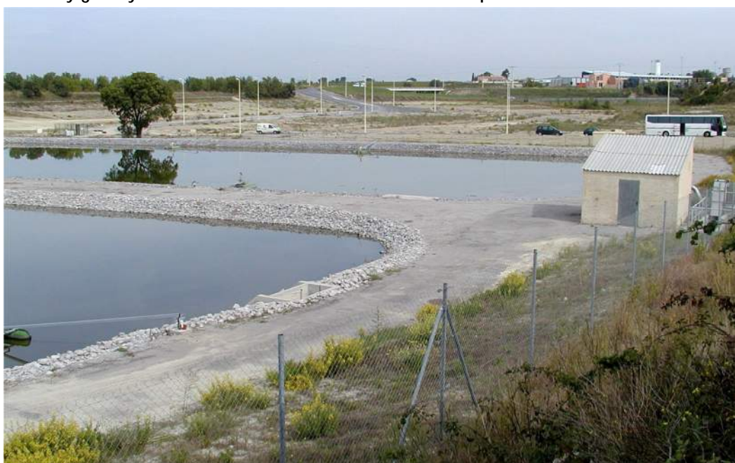
Photo 12: Arrangement of Aerobic Ponds (Dep. Hérault France) (Štencel et al., 2004)
