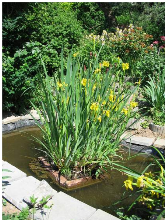
Photo 34: Small Natural Wastewater Treatment Plant without Outflow (Final Treating Tank with Floating Islands with Yellow Iris and Water Hyacinth) Forms an Aesthetic Element in the Garden
