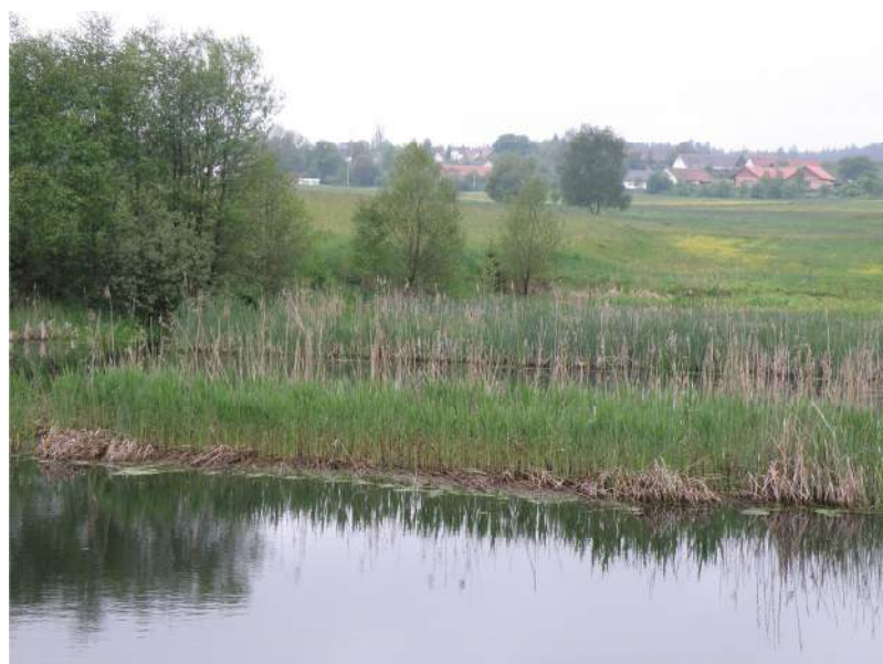
Photo 14: Waste Stabilization Pond with Gravel Shoots Rectifier Planted by Vegetation
