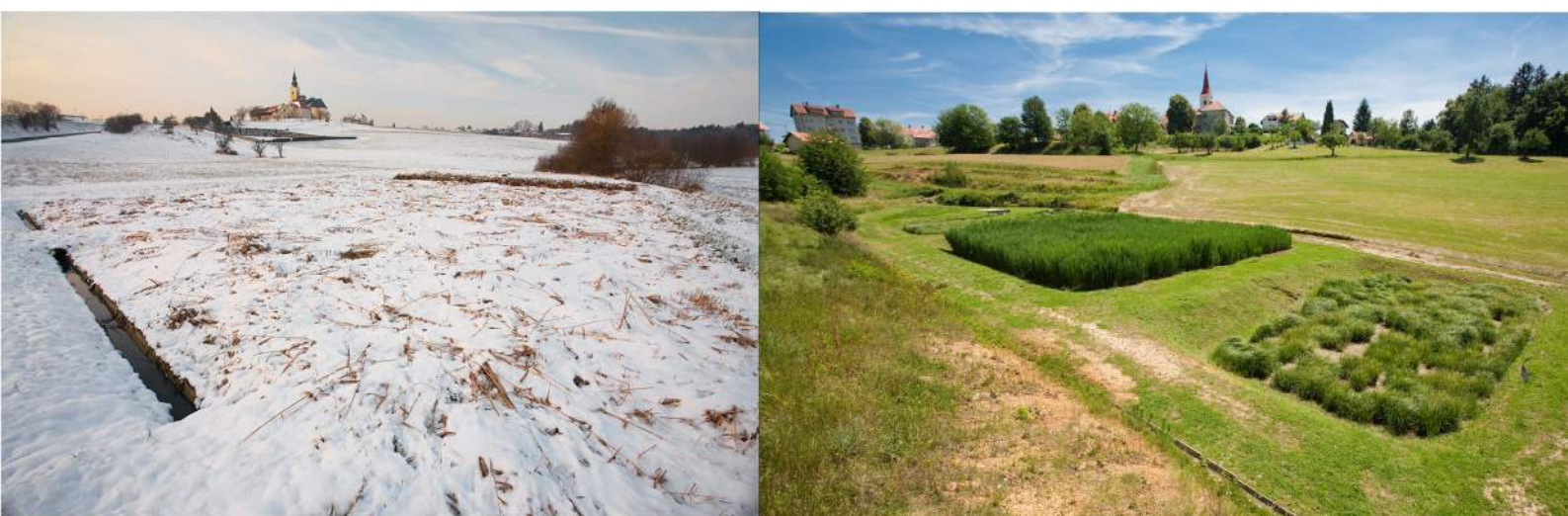
Photo 8: Example of subsurface horizontal flow CTW in Slovenia during winter and summer.
