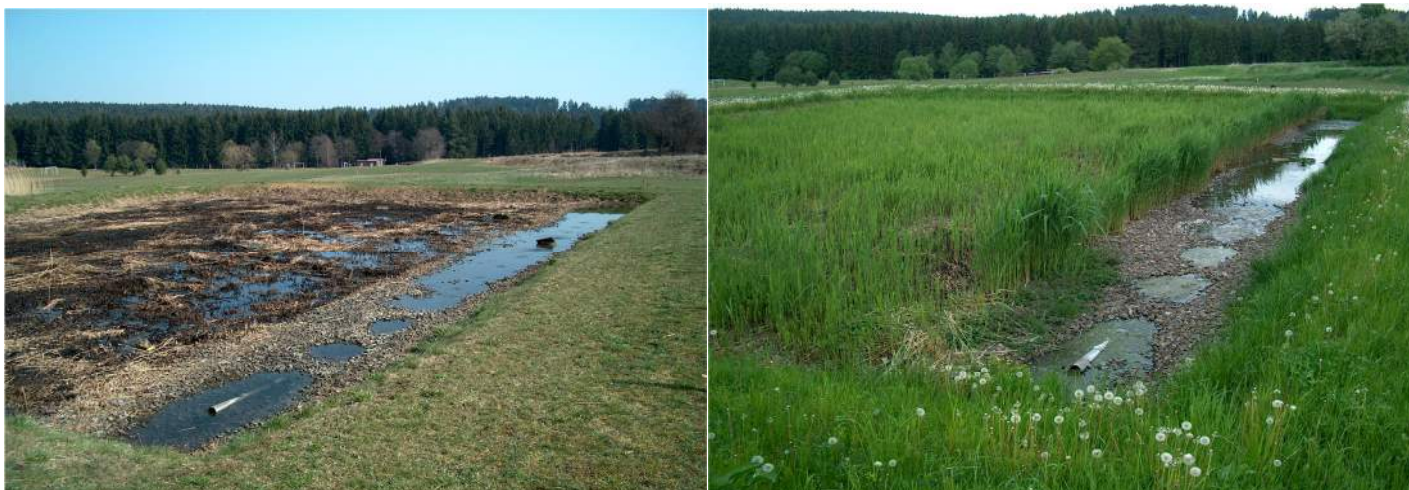
CTW Olší nad Oslavou (CZE) – Vegetation of reed during the growing season (left) - constructed wetland filters after burning of old growth of reed in March – old growth is burned on constructed wetland filters (right)
