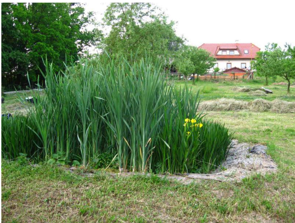
Photo 7: Small Constructed wetland Treatment Plant
