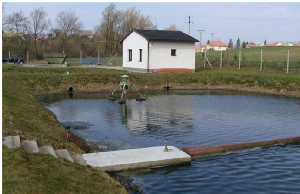
Photo 13: Arrangement of Continuously Aerated Aerobic Pond
