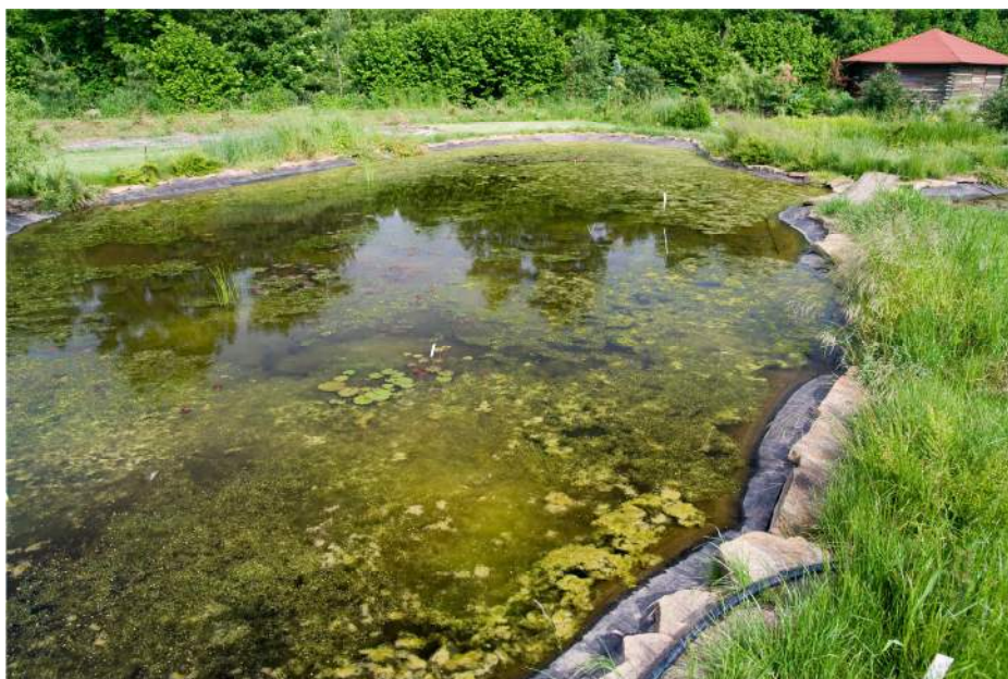
Photo 23: Treatment of water behind the household constructed wetland wastewater treatment plant in the tank with developed aquaculture
