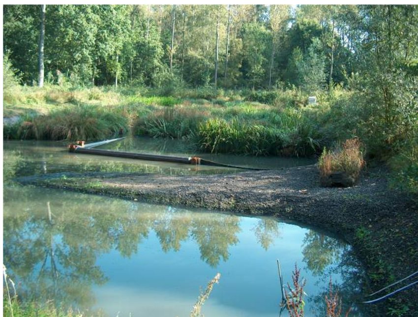
Photo 17: Floating wetland for treatment sewer overflow from a single sewage network in Bornem - Belgium
