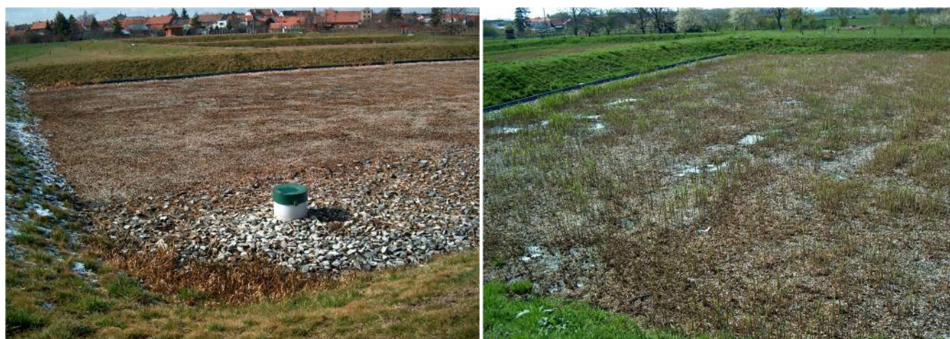
CTW at Čehovice (CZE) – reed during spring period approximately one month after burning old growth (left) – constructed wetland s after burning of old growth of reed in March – old vegetation is burned outside the constructed wetland filters (right)
