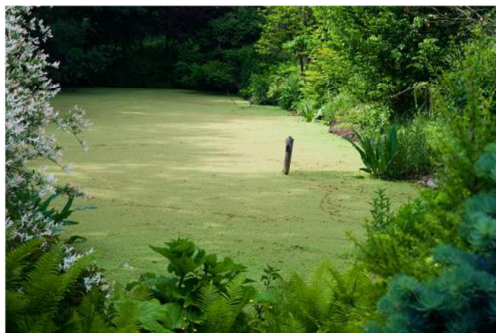
Photo 20: Final treating tank with floating plants on the water surface (duckweed – Lemna)
