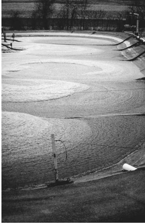
FIGURE 20.3 Concentric circles of different colors and textures of foam due to erratic wasting rates.
