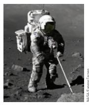
The life-support unit strapped to the back of astronaut Harrison Schmitt weighed 300 lb on the Earth and had a mass of 136 kg. During his training, a 50-lb mockup with a mass of 23 kg was used. Although this strategy effectively simulated the reduced weight the unit would have on the Moon, it did not correctly mimic the unchanging mass. It was more difficult to accelerate the 136-kg unit (perhaps by jumping or twisting suddenly) on the Moon than it was to accelerate the 23-kg unit on the Earth.
