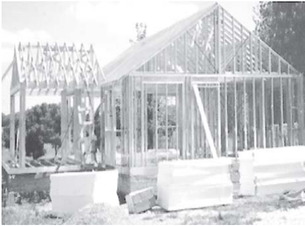
Steel framing is increasingly popular in residential construction.
