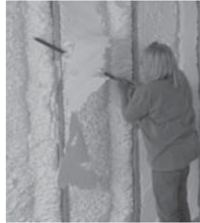
State-of-the-art soft foam insulation is sprayed into walls, floors, and ceilings.
