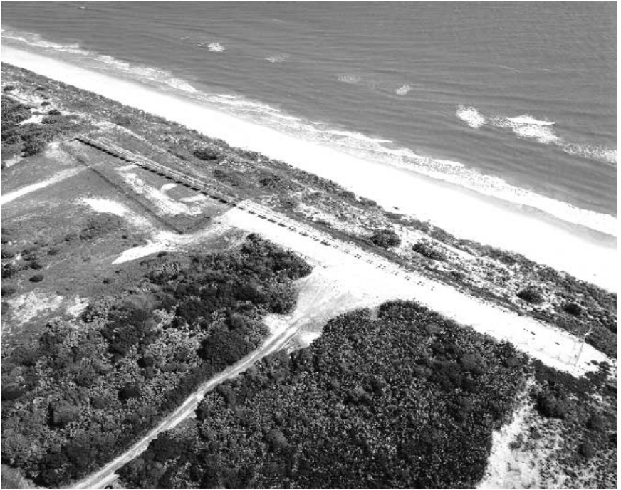
Figure 7.40 Aerial view of the Kennedy Space Center beach corrosion test site.
