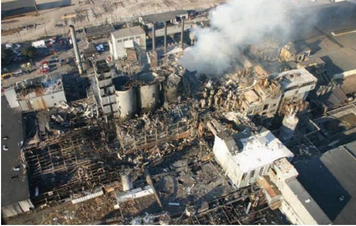
Figure 7.1 Sugar factory after a dust explosion, killing and injuring 50 people [1].
