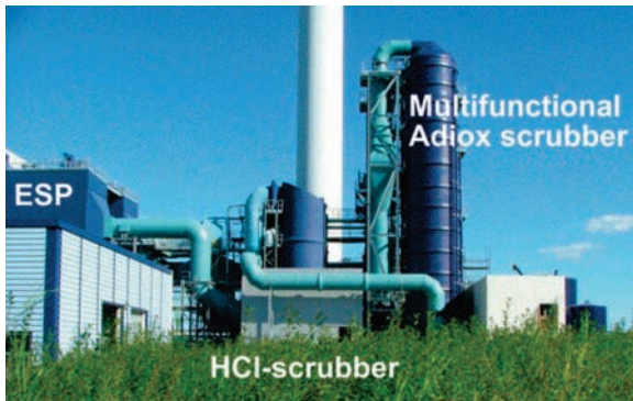
Figure 4.25 Flue gas treatment in a Danish power plant (Måbjergværket). Adiox™ is a process for dioxin removal, see [80] for details.
