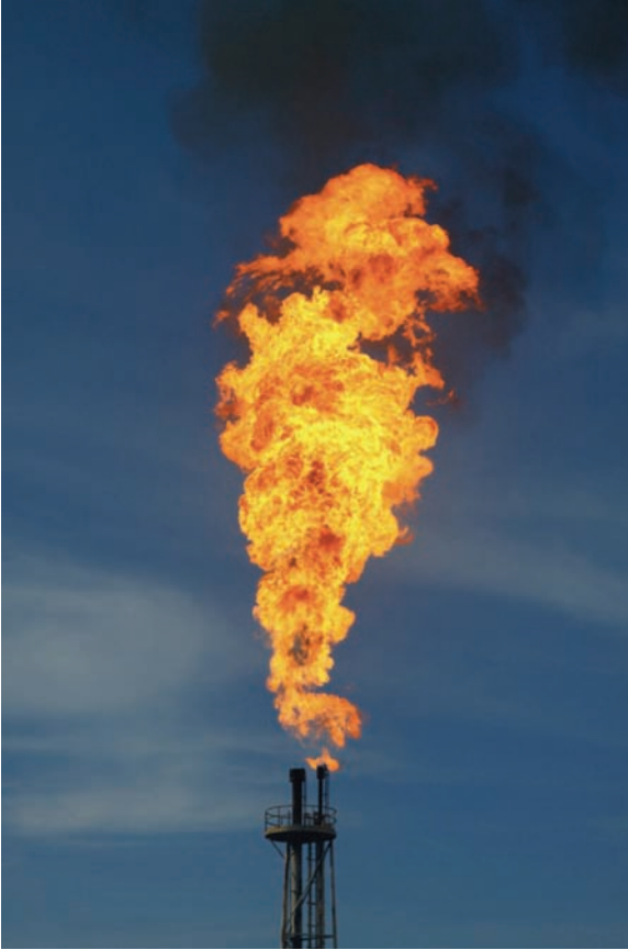
Figure 6.8 Industrial flare for the combustion of waste gases.
