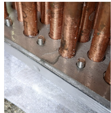
Figure 2.13: Slow leakage in rear manifold sub-assembly.
