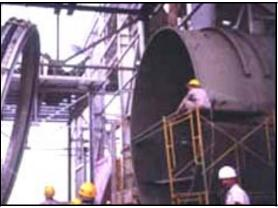
Ø120 inch diameter Gas Turbine Expansion Joint during installation. 25 in wc at 1070°F.
