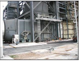
GT Diverter Bypass System for Alstom GT13E2 in Greece
