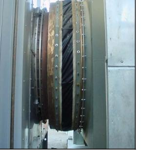
Ø89 inch diameter Gas Turbine Exhaust Expansion Joint with Hot to Cold Frame. 25 in wc at  $980^{\circ}$ F.
