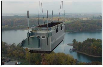
SCR 4-port diverter module being lifted into place in the United States
