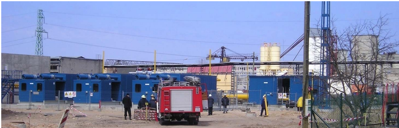
Start-up of three (3) gas booster compressors.
