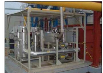
Above three extended gas skids with KO-vessel, 2x 100% particle and 2x 100% coalescing filter, electric heater (with thyristor control panel), stainless steel piping & vessels and a flow meter
