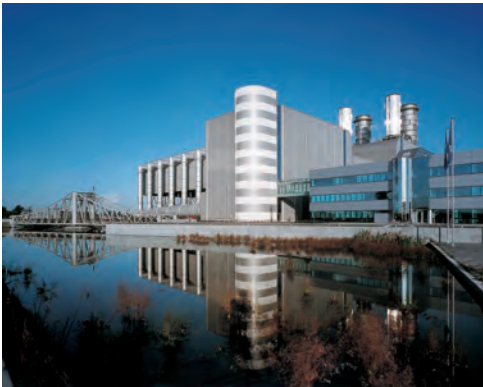
460 MW Combined Cycle Power Plant Bruges, Belgium
