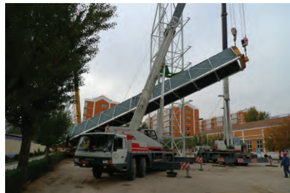
A 25m high MegaDelta being lifted
