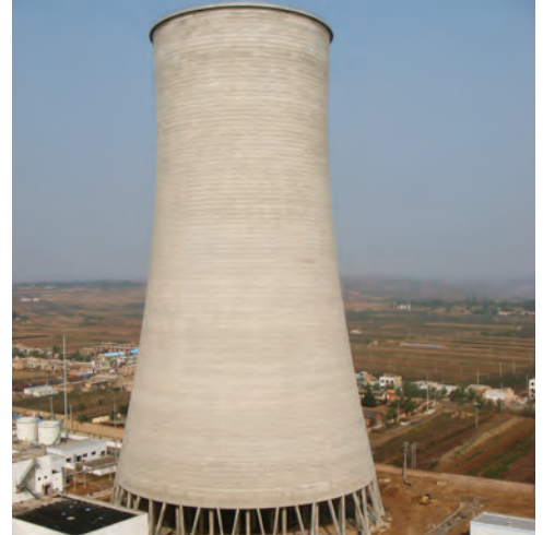
Coal Fired Power Plant – Auxiliary Cooling System Tongchuan, China – 2006
