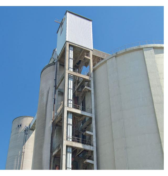
Bucket Elevator for cement silo feeding
